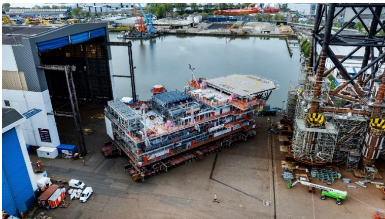
Production platform N05-A under construction
