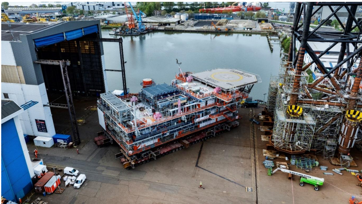
Production platform N05-A under construction
