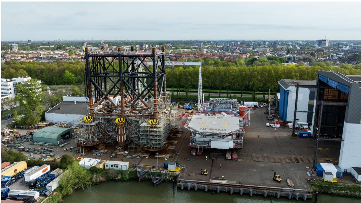
Production platform N05-A under construction
